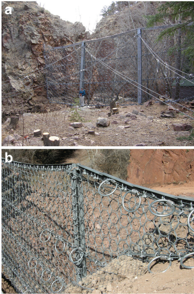
Fig. 3. (a) Upper fence with person for scale; (b) Fence showing rings and smaller mesh with 113 mm opening. Photos taken 7 April 2013.
