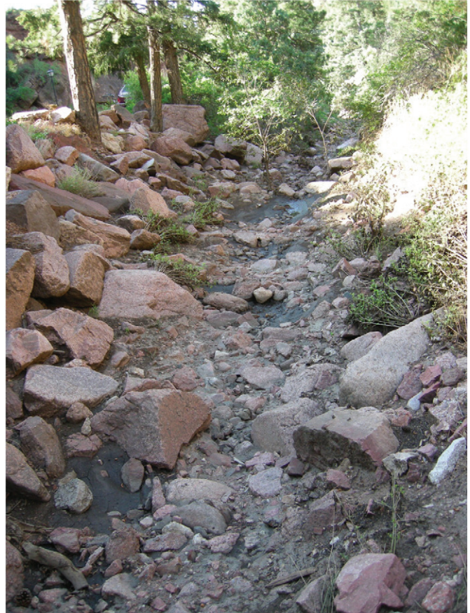
Fig. 6. Channel character downstream of lower fence before construction.
