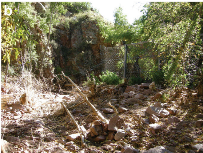
Fig. 5. Upper fence blocking particles from transport downstream. Photos taken 3 October 2013.
